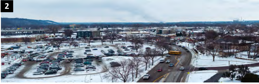
Conflicts between student parking, drop-off/pick-up activity, and access points exist at this entrance.
