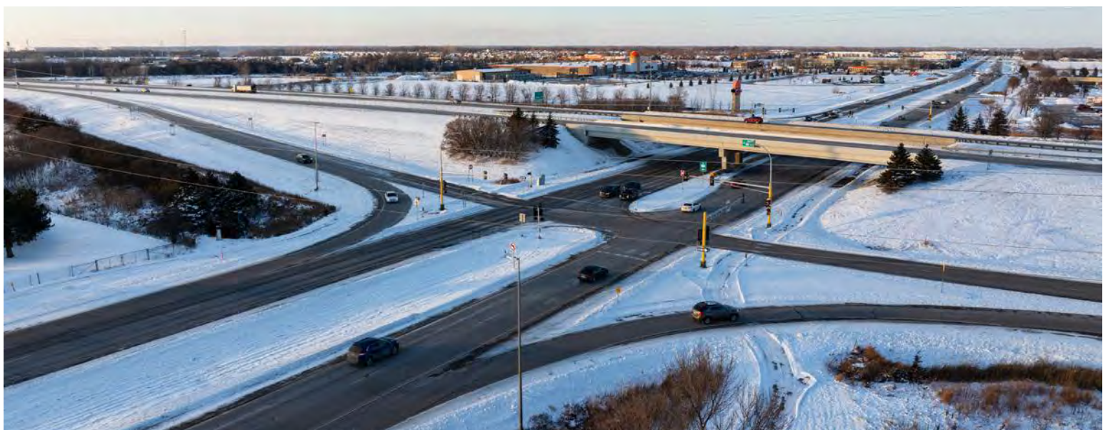
Existing Highway 14/22 interchange
