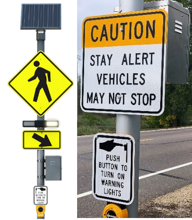
Posted mounted, solar powered RRFB (right); Example of additional warning signage for the RRFB user, created in collaboration with SRF and Dakota County to provide extra warning before crossing (far right).
