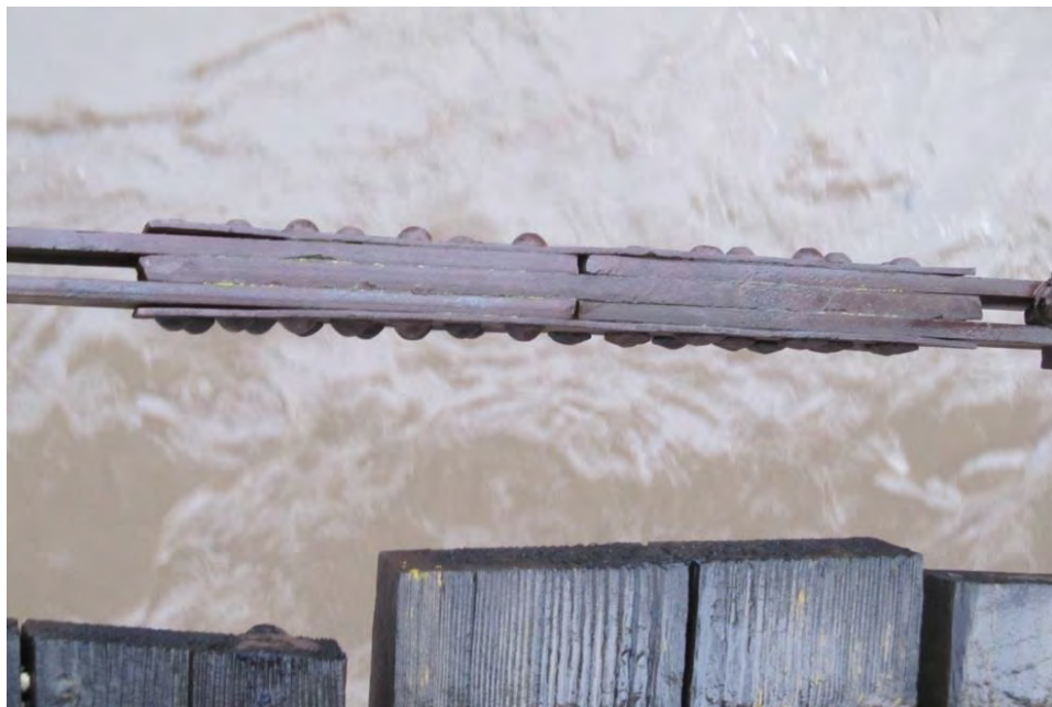
Photo 7: Bottom chord showing distortion of splice plates
