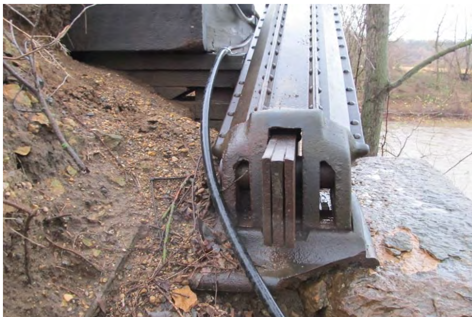
Photo 16: Bearing at east abutment
