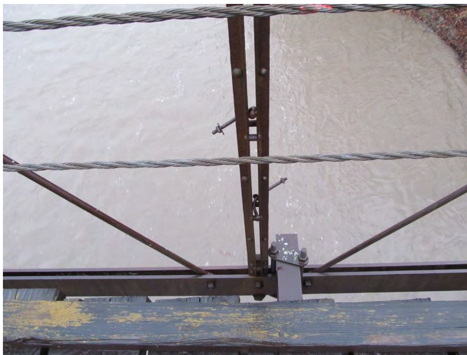
Photo 10: Typical built-up vertical member (note previous railing hardware remaining)
