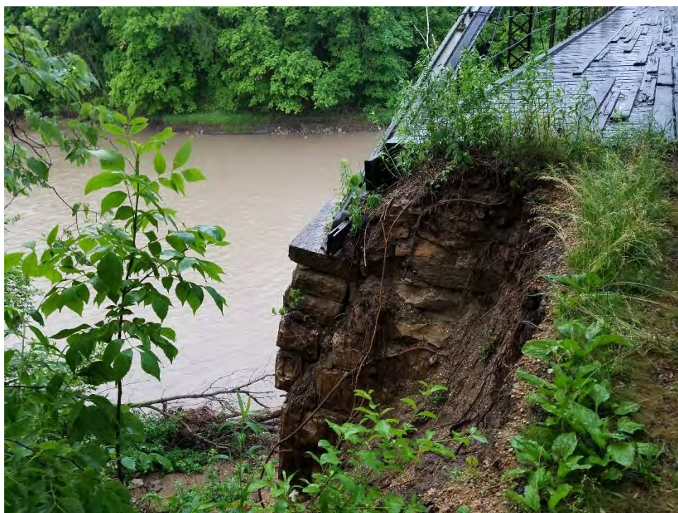
Photo 24: Southeast slope washout, exposed stone masonry abutment
