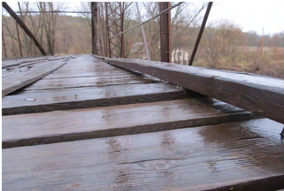
Photo 15: Timber deck (note uneven surface, potential tripping hazard)
