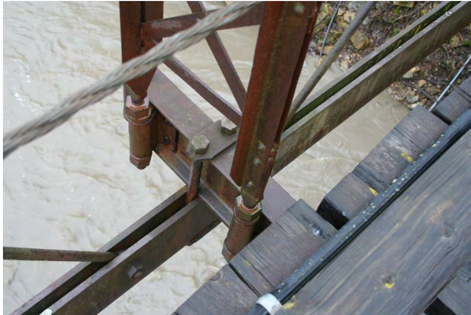
Photo 21: Typical bolted connection, vertical to bottom chord
