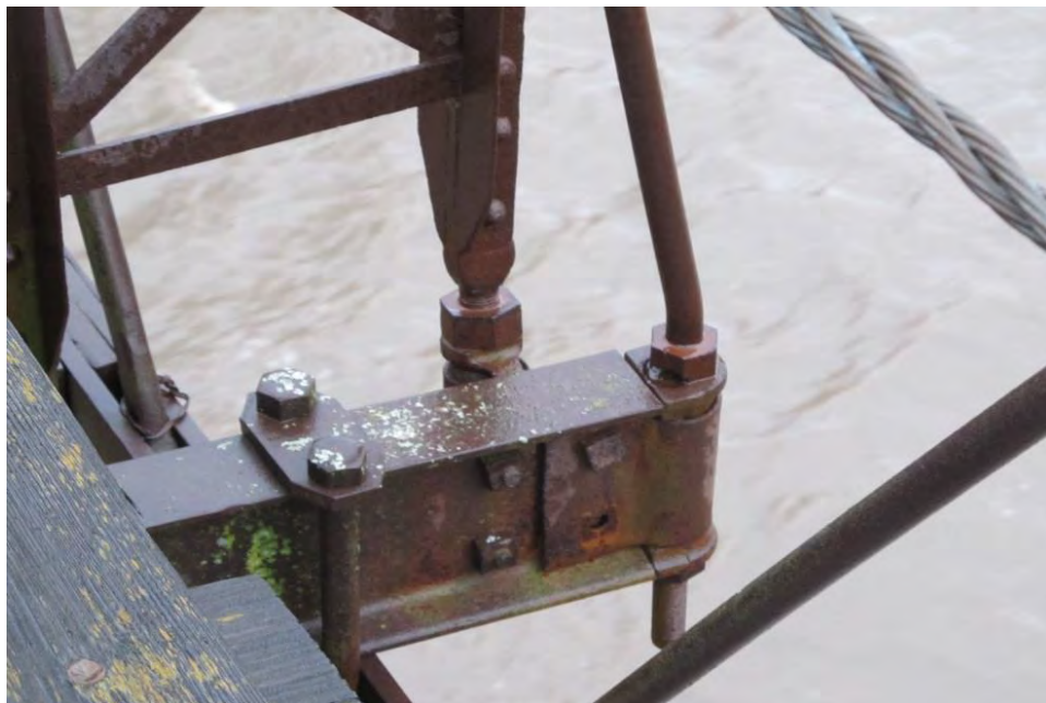
Photo 13: Missing bolt at secondary member connection (1 of 2)
