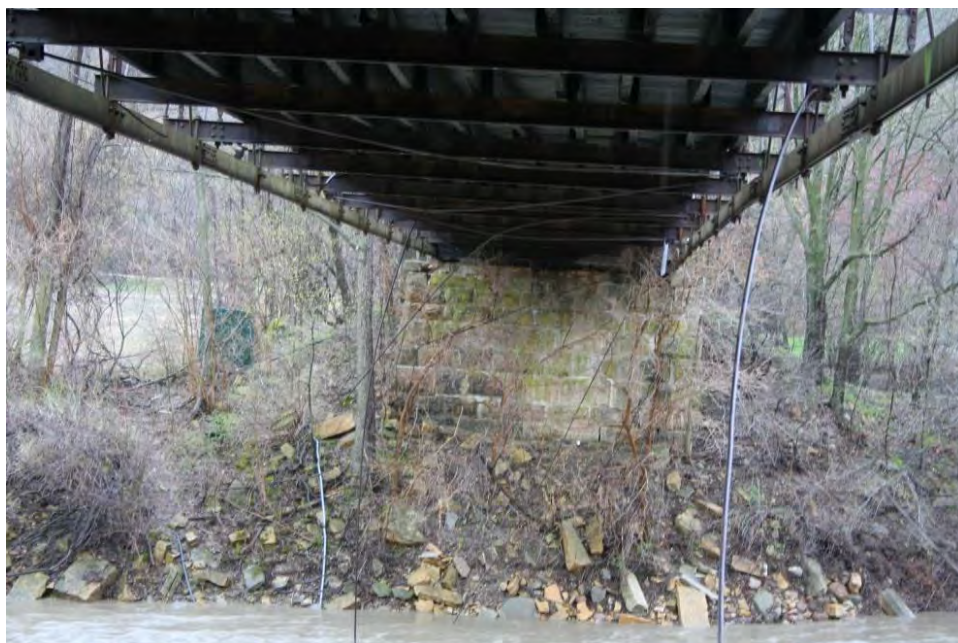
Photo 12: Floorbeams and timber stringers (note hanging X-bracing)
