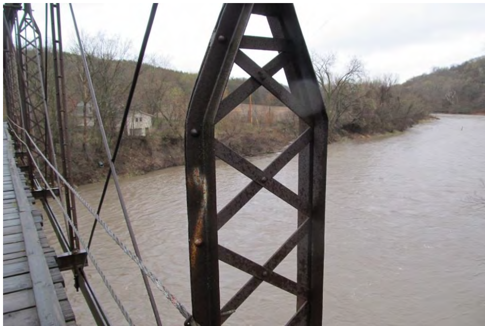
Photo 9: Typical latticed vertical member
