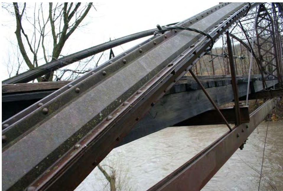
Photo 8: Top chord configuration (Phoenix Column)
