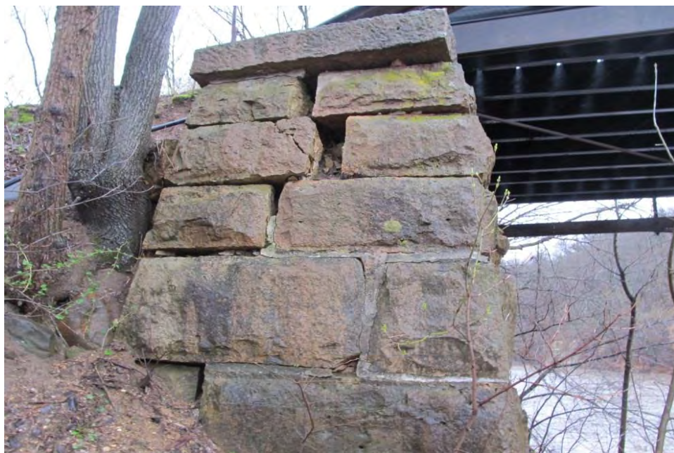
Photo 18: East abutment masonry dislocation, northeast corner
