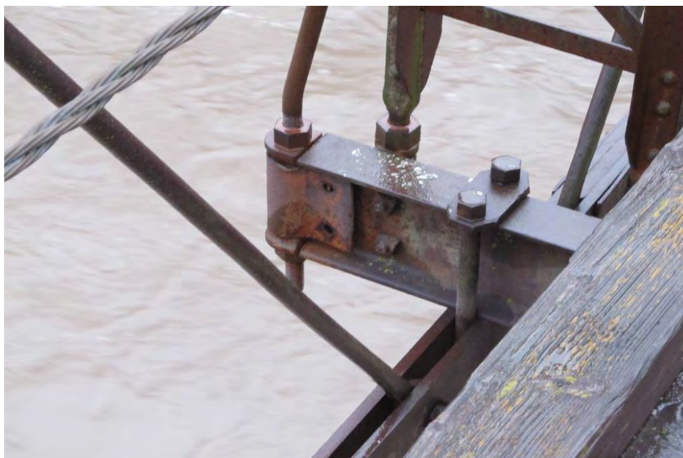
Photo 14: Missing bolts at secondary member connection (2 of 2)
