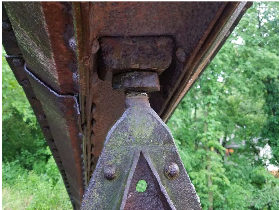
Photo 22: Typical bolted connection, vertical to top chord
