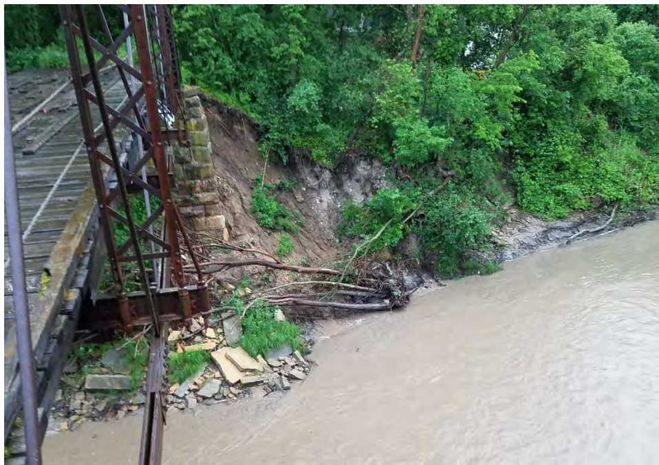
Photo 23: Southeast slope washout
