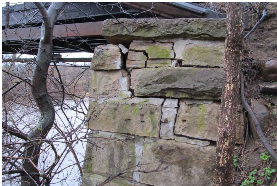
Photo 17: East abutment masonry dislocation, southeast corner
