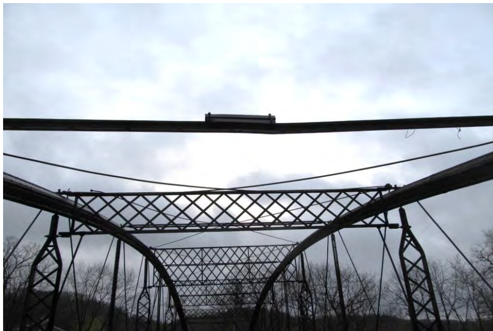
Photo 11: End portals and sway braces
