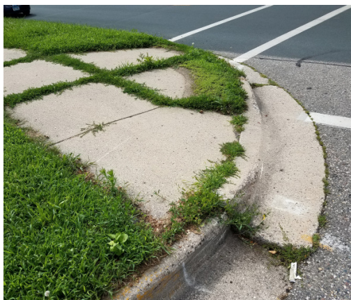
A non-compliant pedestrian ramp with vertical discontinuities greater than 1/2 inch, vegetation growing through cracks, and no detectable warning such as truncated domes.
