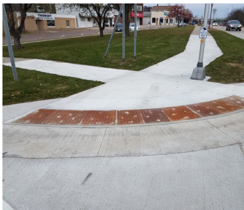
An ADA-compliant, blended transition or fan, pedestrian ramp with truncated domes and easy access to the pedestrian access route.
