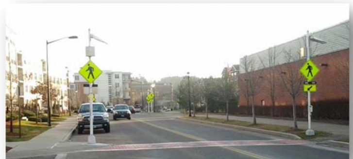
Figure 18. Ground-Mounted Rectangular Rapid Flashing Beacon
